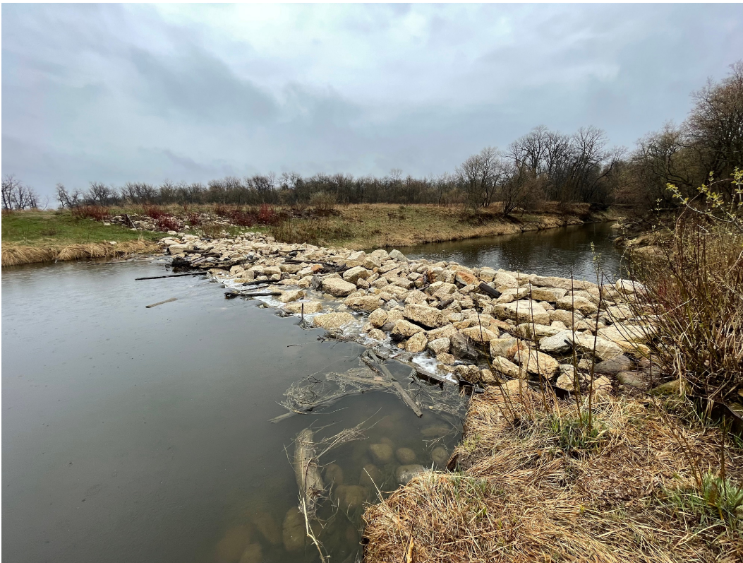
Figure 3. Boyne River at McEachern Bridge site, May 2, 2024, discharge approximately 1.2 CMS: (a) looking upstream toward existing timber bridge remnants; (b) looking northeast along sheet-piling weir with angular riprap, i.e., the McEachern Dam (photos: Samson Engineering 2024).
